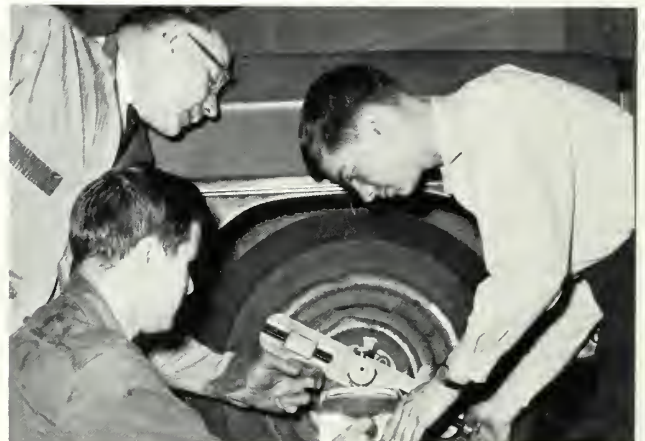
Delicate front-end adjustment being performed on a late model vehicle.
